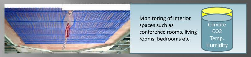
Innovative capillary tube mats or other area cooling systems can be used to provide an optimum heating and cooling system for ceilings, floors and walls. The sensor module ensures the recording of the physical parameters and controls the states of the control. It can also be used for a quick and precise detection of CO2 concentrations.
